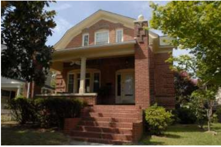
One of the many Sears houses is shown that was shipped by rail car to Cape Charles as a building kit. A tour of several of the kit houses in Cape Charles will be Saturday. / JAY DIEM/THE DAILY TIMES
